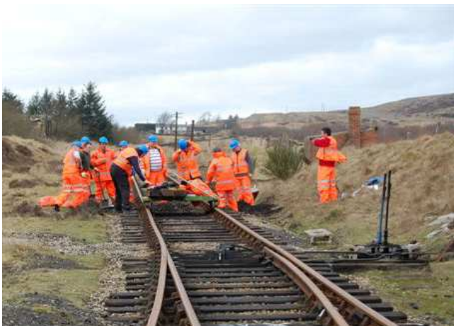
Above—The Greenlight trainees replace sleepers on the main running line. Andy May
