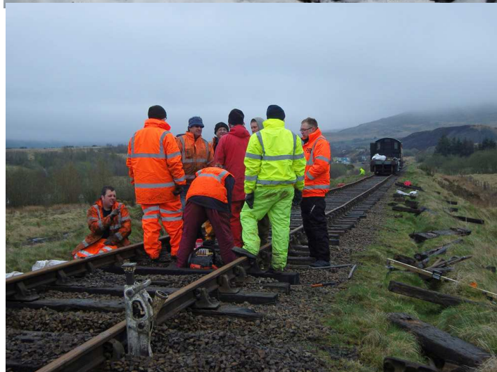
Above—The Greenlight trainees replace sleepers on the main running line. Andy May
